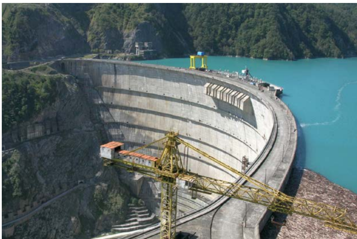
Fig. 20. Zapora i elektrownia wodna Enguri Fig. 20. Enguri dam and hydroelectric power plant
