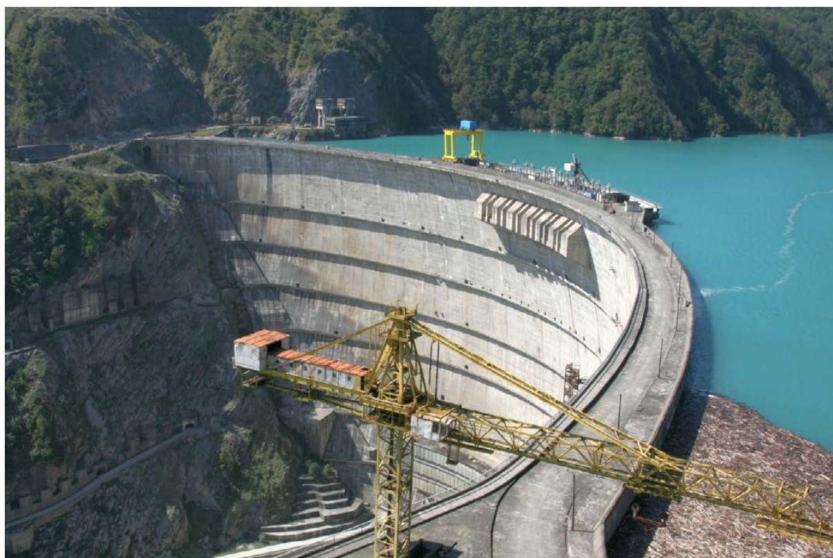
Fig. 20. Zapora i elektrownia wodna Enguri Fig. 20. Enguri dam and hydroelectric power plant
